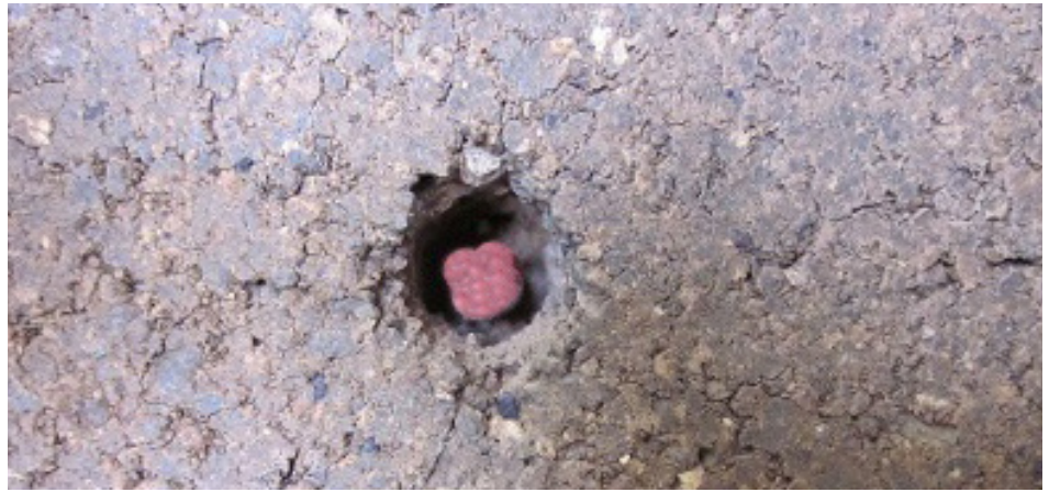
9mm CD Tie installed using SDS countersunk CD Tie Tool Note: the red tip of the 9mm CD Tie unique to Thor Helical indicating 316 SS
