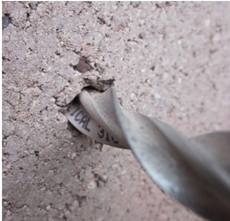
CD Tie installation
