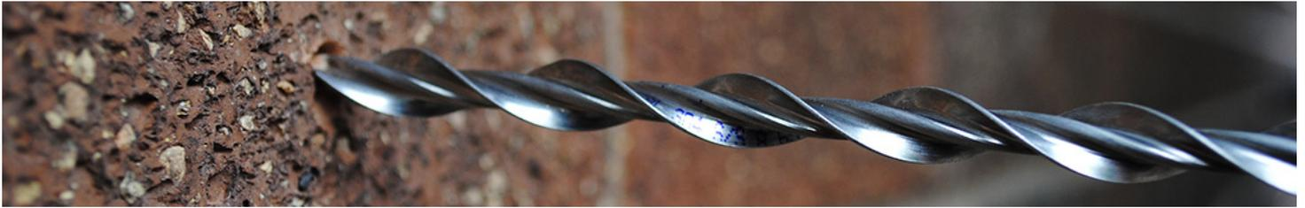
Replacing cavity wall ties with a remedial tying system is a low-cost alternative to rebuilding walls that are suffering from wall tie corrosion. For 30 years wall tie replacement has become the accepted method of solving the problem of cavity tie failure.
